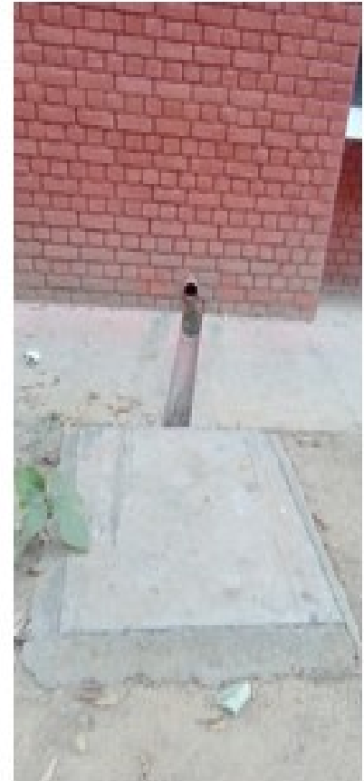
RAINWATER TRAP UNIT (3 ft x 3 ft x 3 ft)
