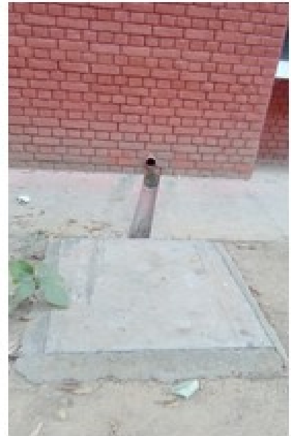
RAINWATER TRAP UNIT
